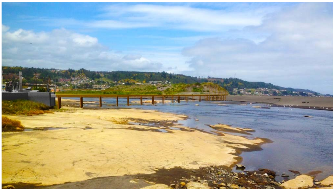
PELLUHUE TRAMO 1 SECTOR PASARELA
