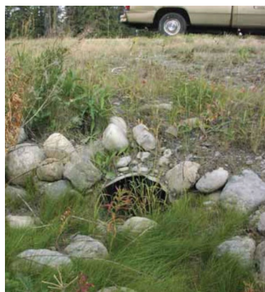
Paso para pequeños mamíferos y anfibios. Fuente: Wildlife Crossing Structure Handbook Design And Evaluation In North America (Central Federal Lands Highway Division, 2011)
